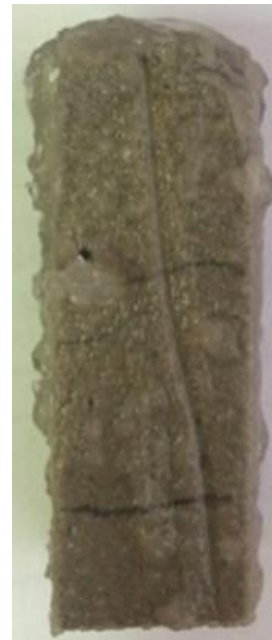
Fig. 4. Acid corrosion of set cement.
